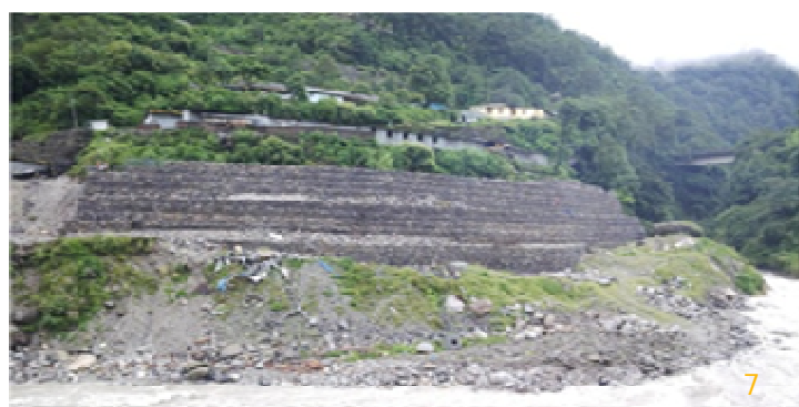
Photograph 6 & 7 : Lachen chu Right Bank Maccaferri Treatment
