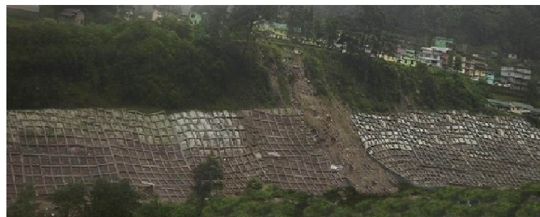
Photograph 8: RCC Grid Beam Treatment on Lachung Right bank
